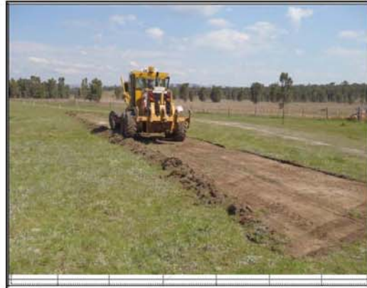
Description: grader scrape of the carpark crib shed loca
