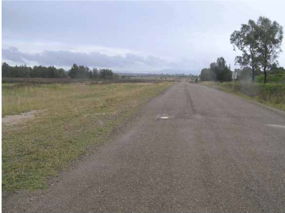
Figure 7 Sealed section of Brunkers Lane.
