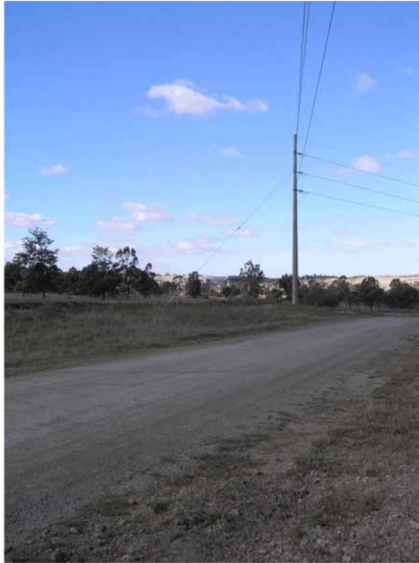
Figure 8 Unsealed access road on Macquarie Generation lease.
