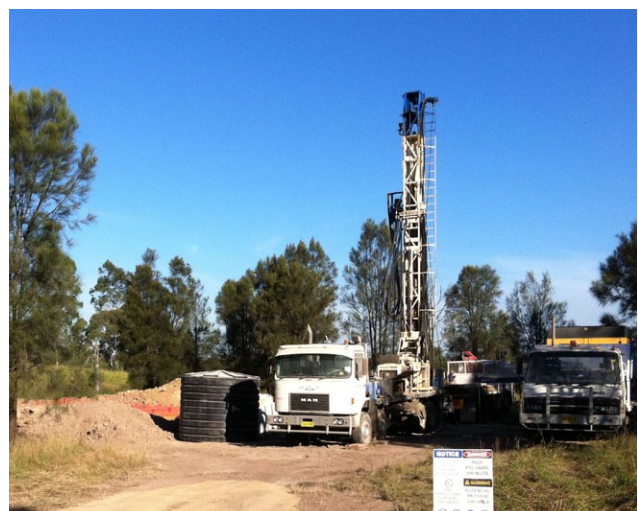
Figure 6 (top): Small pad with a gas bore (5 x 5 m compound) for bores that are connected to the central gas drainage plant (Source: ACOL)
