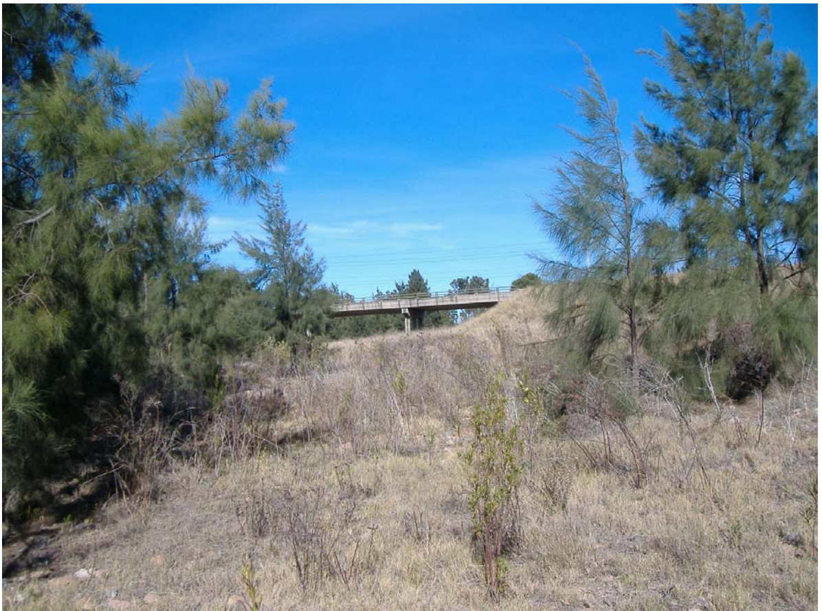
Photograph 2 Proposed pipeline route looking along north bank of Bowman's creek; toward New England Highway Bridge
