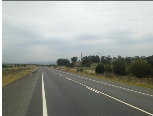
Figure 5 Lemington Road looking South
