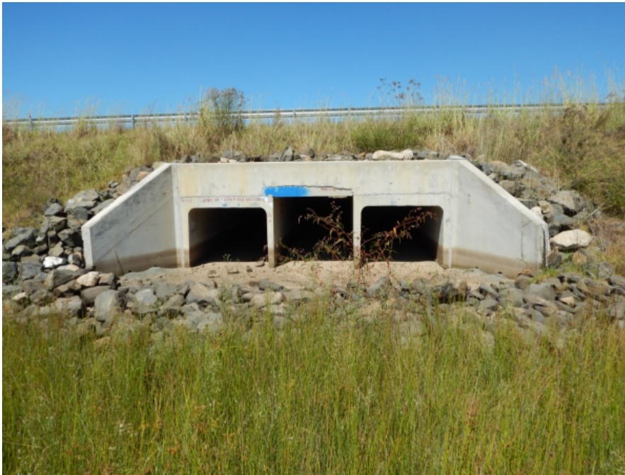
Plate 2: Lemington Road northern Culvert
