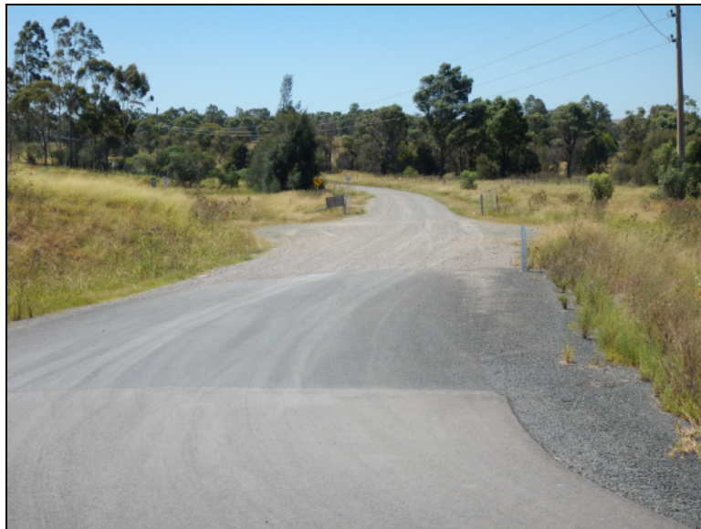
Plate 1: AGL Macquarie South Access Road Looking North from Lemington Road Intersection
