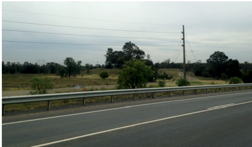
Plate 1: 33kV Transmission Line Adjacent to AGLM South Access Road
