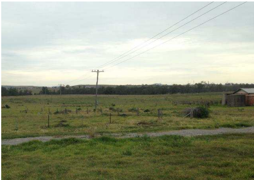
Plate 2: 11kV Ausgrid Transmission Line above Longwalls 5 and 6
