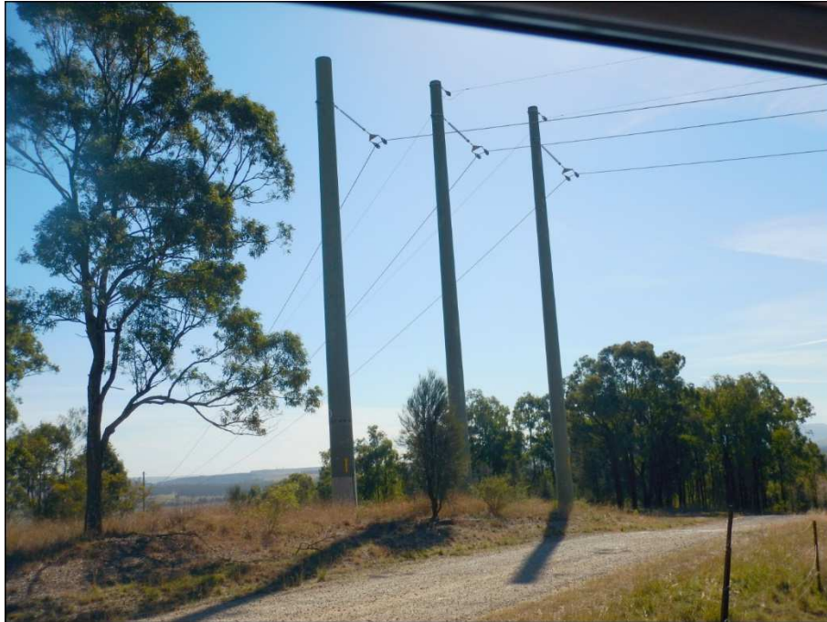
Figure 2: Set 24 (with conductor sheaves) at change of direction.
