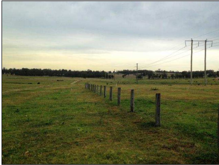
Plate 1: Southern 132kV Ausgrid Transmission Line Looking East from Last Two Pole Timber Set
