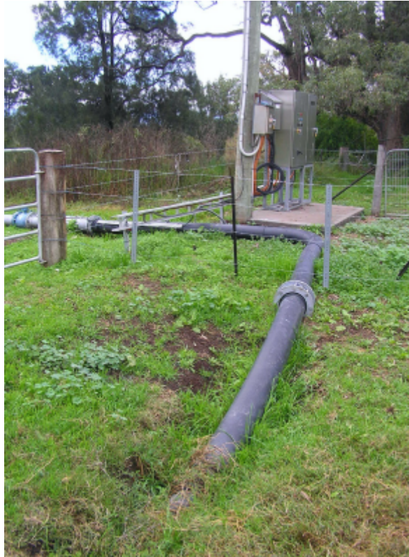
Plate 2. ACOL Water Supply Pipeline
