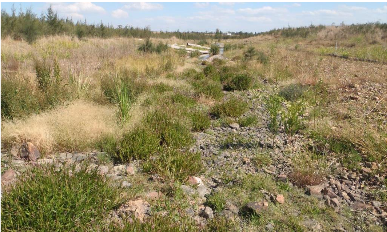
Photo 1 Eastern Diversion Looking Downstream
