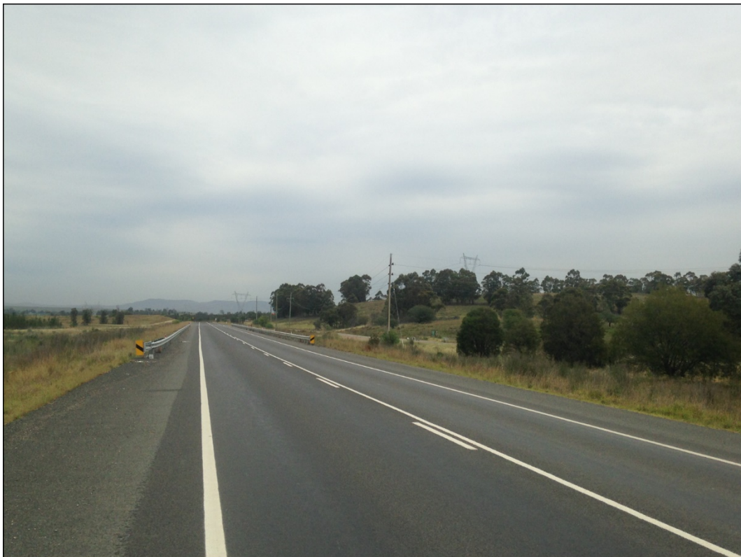
Figure 7: Lemington Road looking south.
