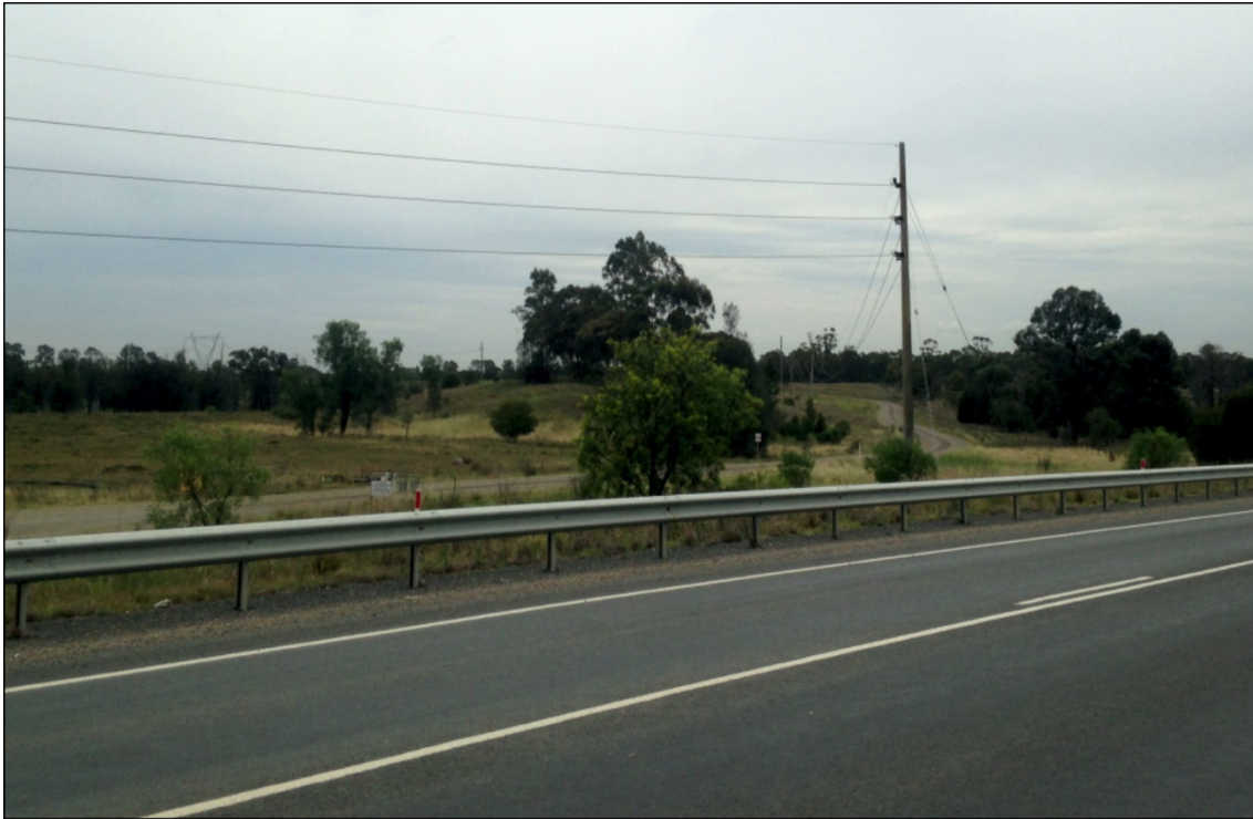
Figure 13: 33kV Powerline adjacent to AGLM south access road.
