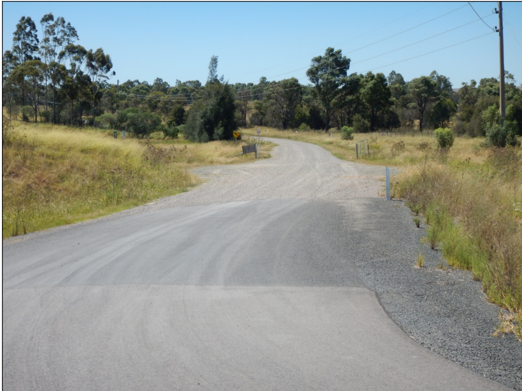
Figure 14: AGLM south access road.
