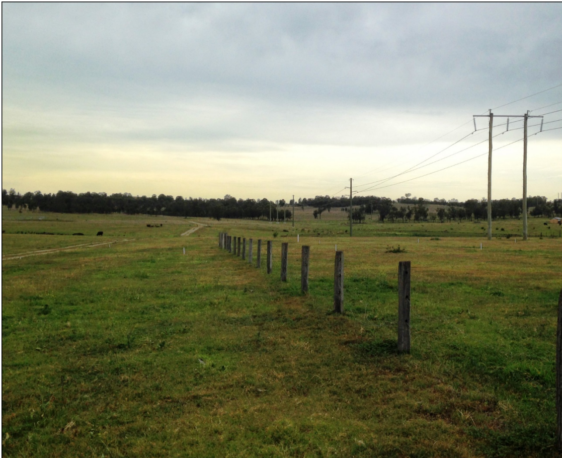
Figure 11: Southern 132kV AusGrid Powerline.
