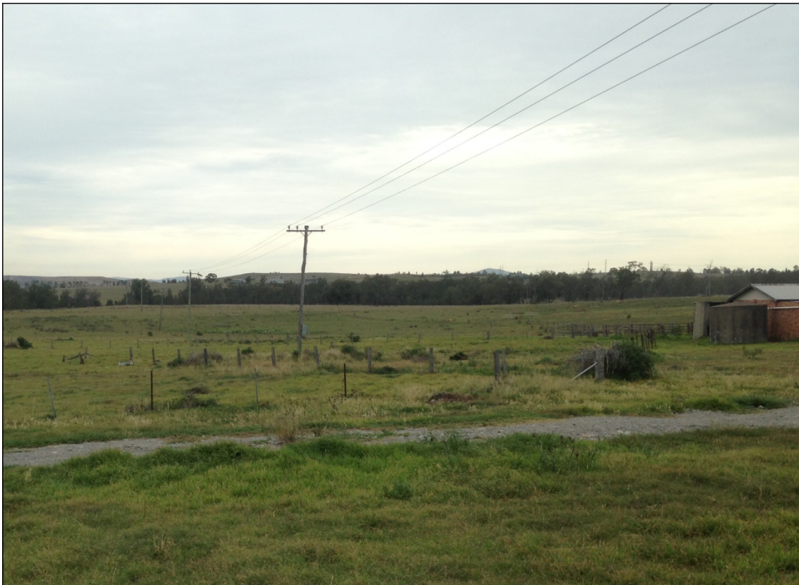
Figure 12: 11kV AusGrid Powerline above Longwall 5.
