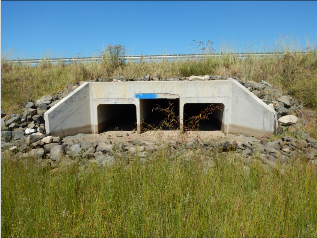
Figure 9: Lemington Road northern Culvert.
