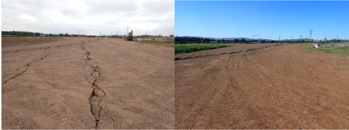
Photo 2: Example of subsidence cracking along stacked goaf edge and after crack remediation
