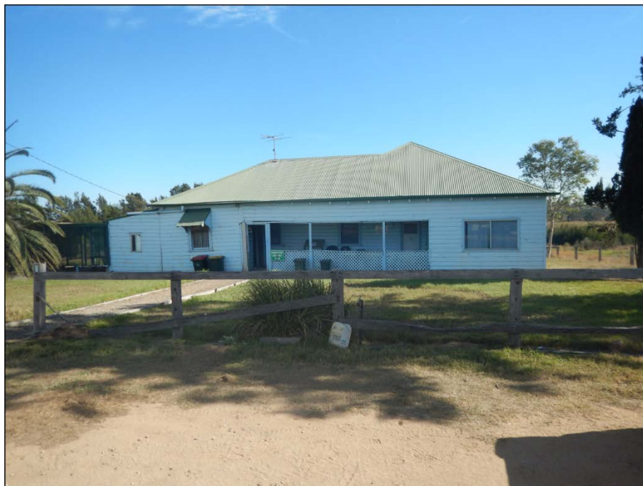
Figure 14: Residential structure 'Ashton' located to west of Longwall 204.
