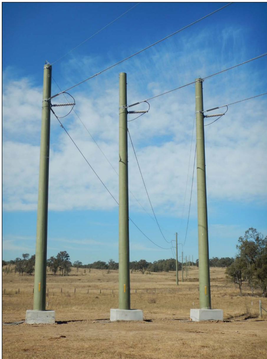
Figure 12: 132 kV powerline that traverses the southern end of Longwalls 201-204.
