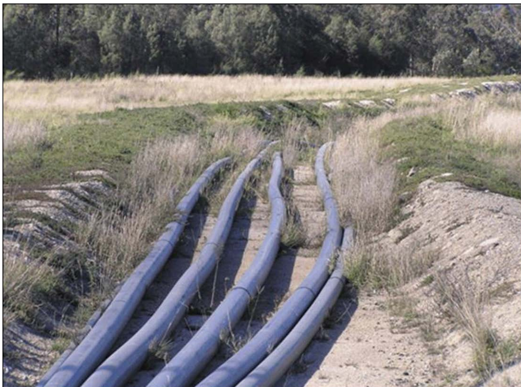
Figure 21: ACOL tailings disposal lines in open trench.
