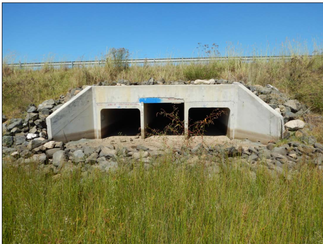
Figure 12: Lemington Road Culvert.
