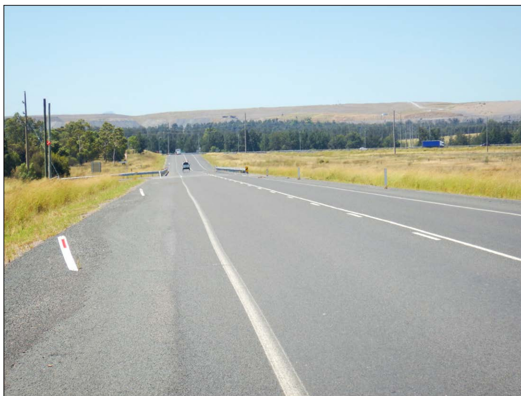
Figure 10: Lemington Road looking north from about CH1000m with AGLM Access Road evident in the middle distance and the culvert midway along the barriers. Traffic on the New England Highway is evident in the distance.
