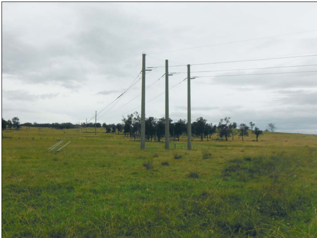
Figure 15: 132kV AusGrid Power Transmission Line.
