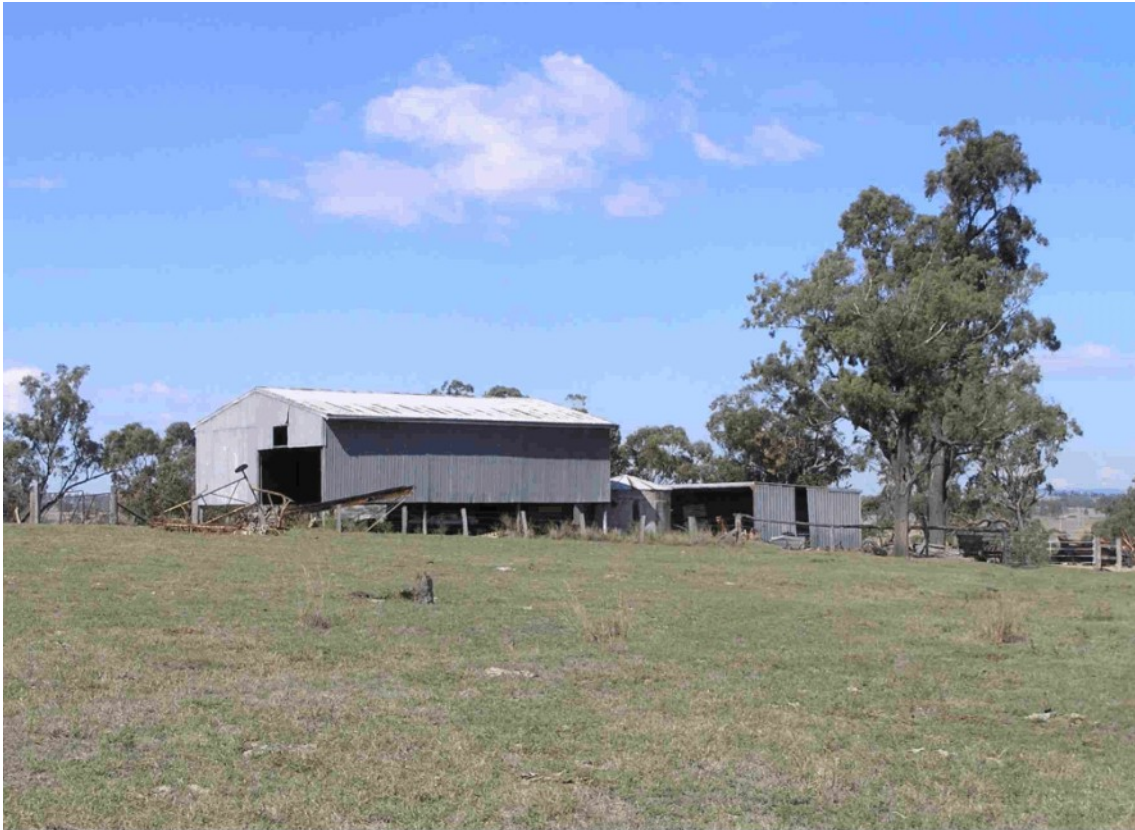
Figure 17 Photograph of farm buildings on Property 130 located within the SMP Area.
