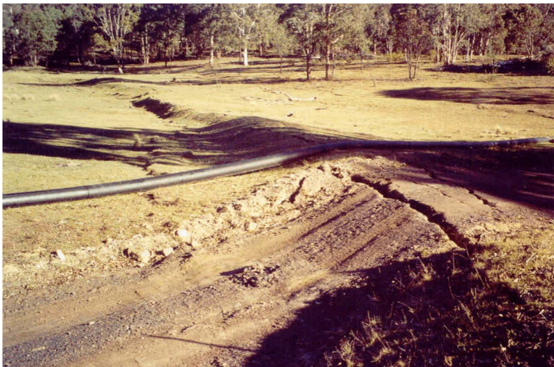
Figure 25 Example of post-mining compression hump at 60m overburden depth.
