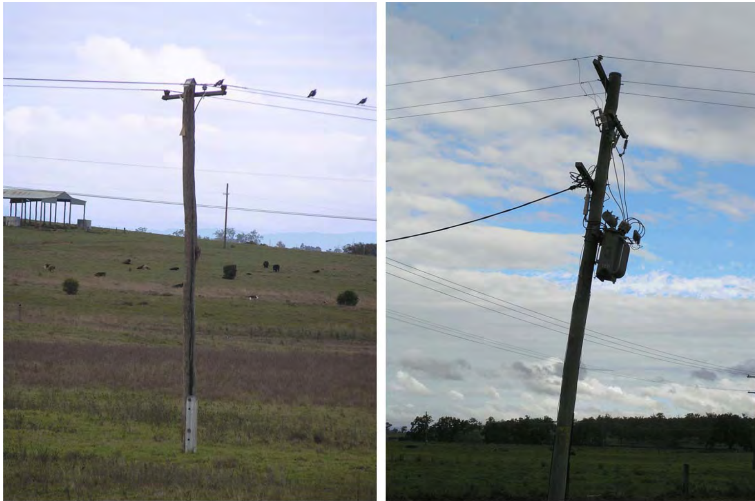
Figure 11 Photographs of single pole structures on local electricity lines.
