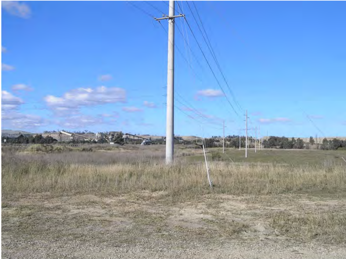
Figure 7 Photograph looking east along New England Highway road reserve.
