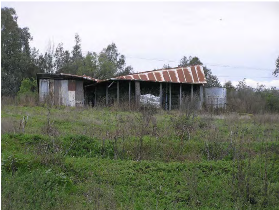
Figure 19 Disused shed beyond the northern end of Longwall 9.
