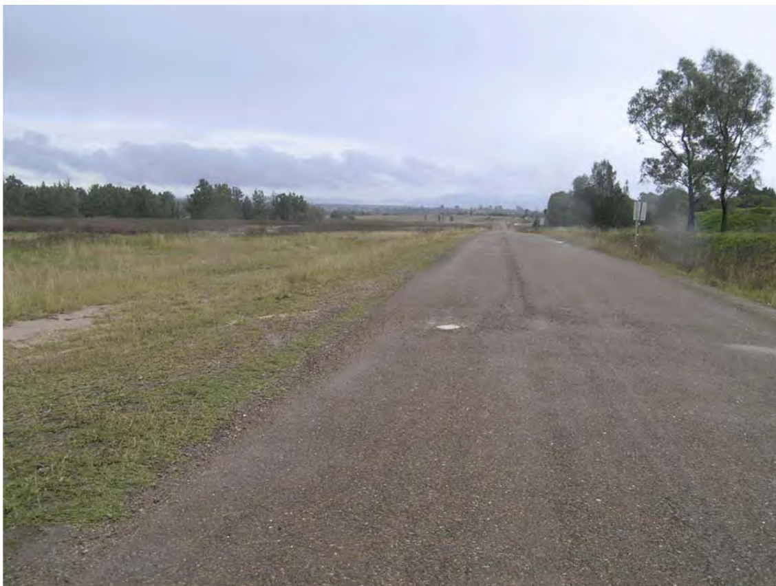
Figure 13 Sealed section of Brunkers Lane.
