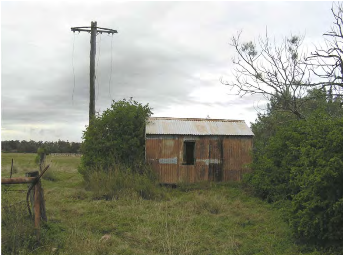
Figure 18 Disused pump shed adjacent to Bowmans Creek.
