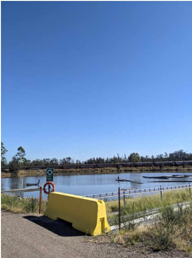
Plate 4.1 Process water dam
