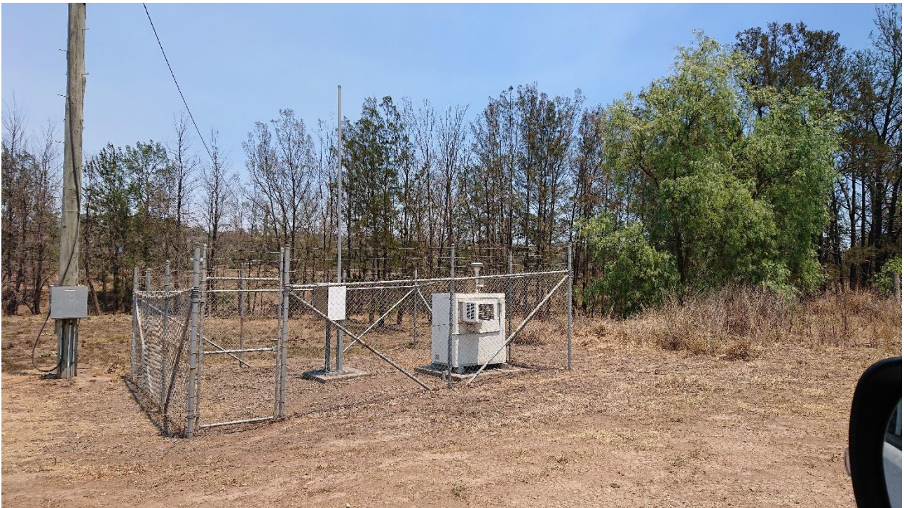
Photo # 1 - Air Quality Monitoring Station
