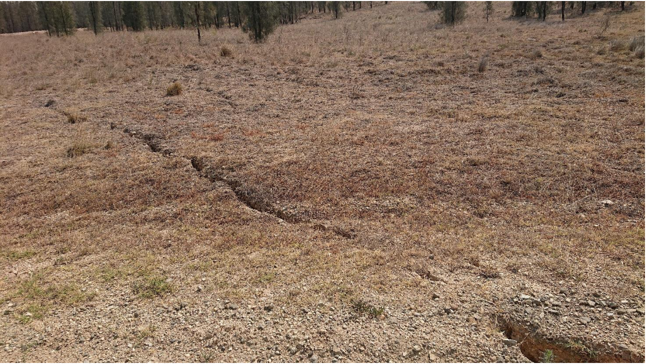
Photo # 6 - Subsidence Cracking
