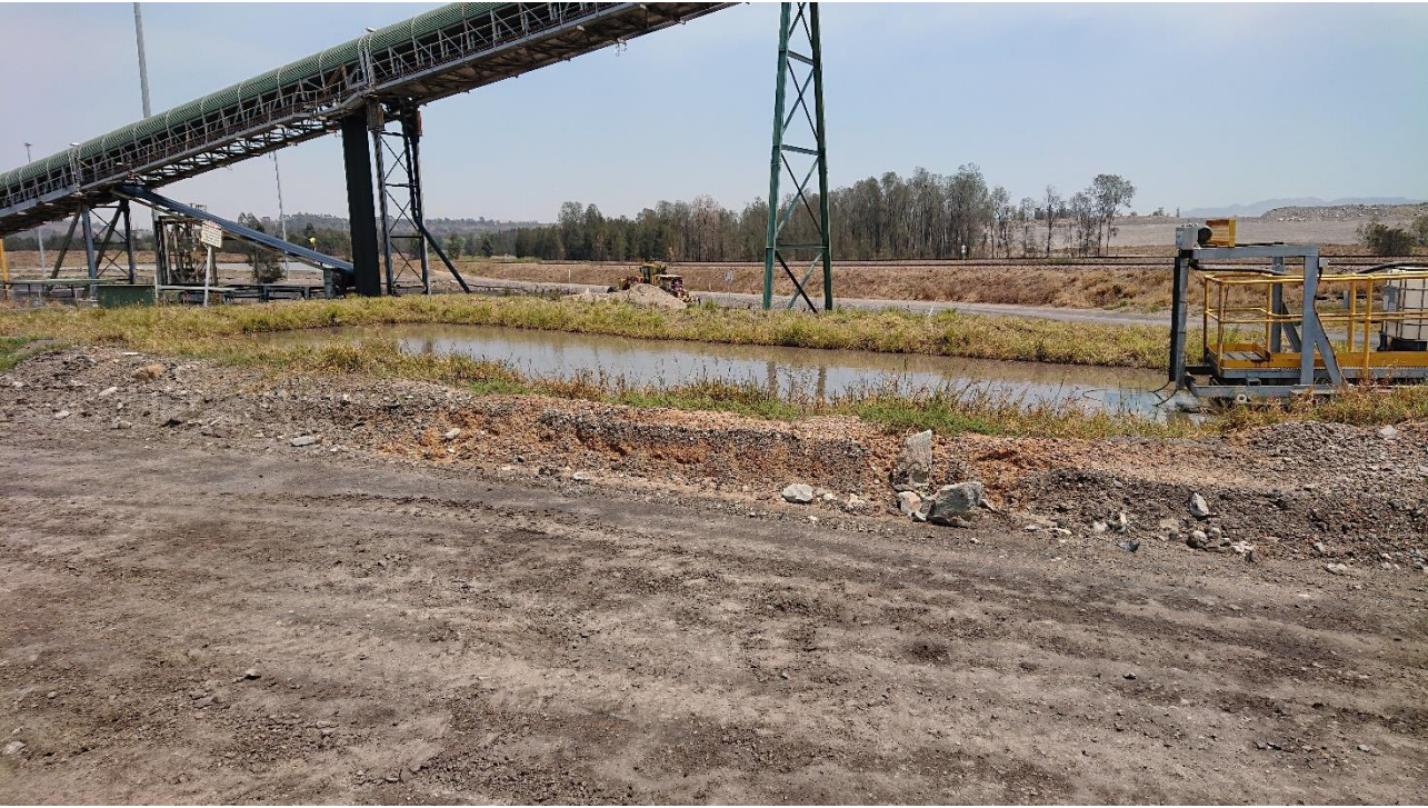
Photo # 14 - Sediment Pond with oil / water separator
