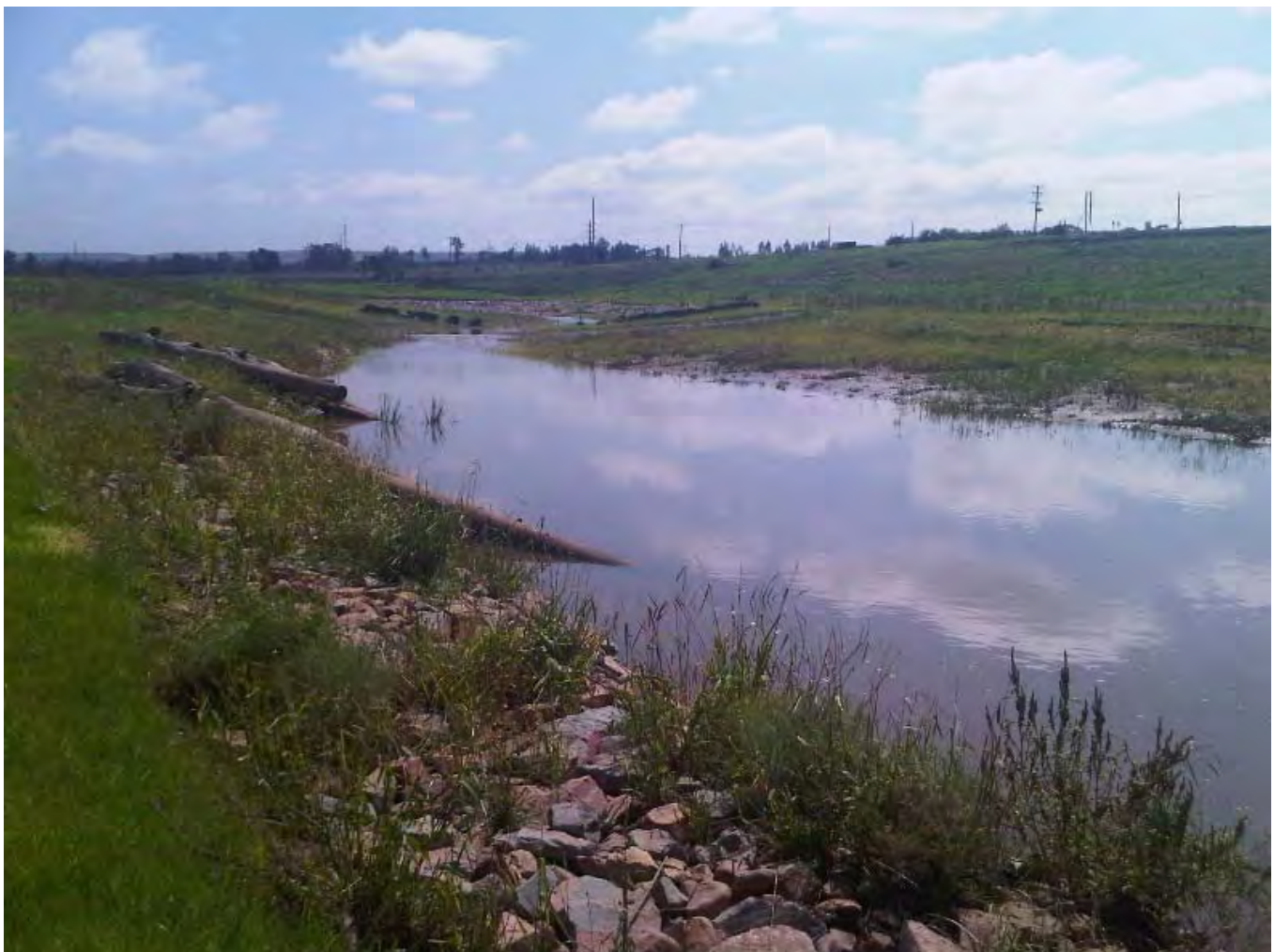
Bowmans Creek Diversion
