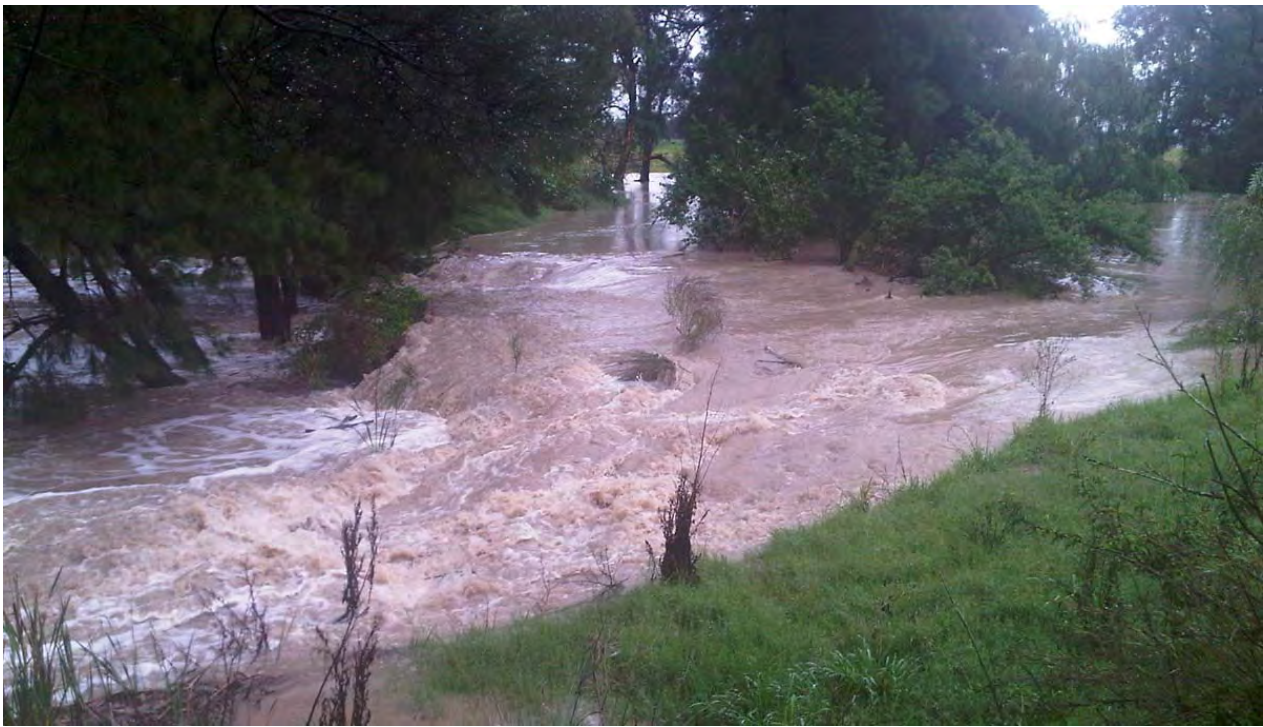
Figure 23: Connecting channel between EDC and Bowmans Creek in flood January 2013
