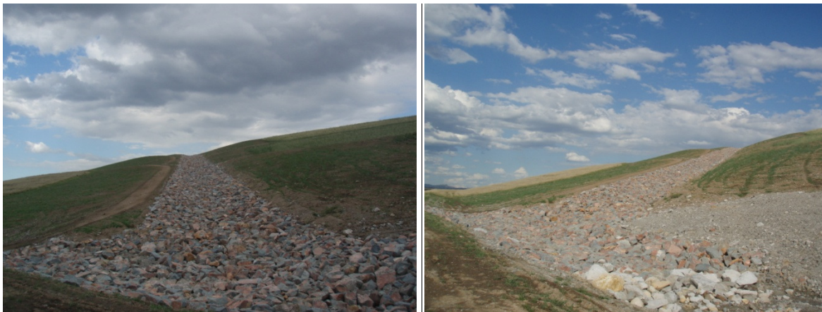
Figure 35. Northern drop structure
