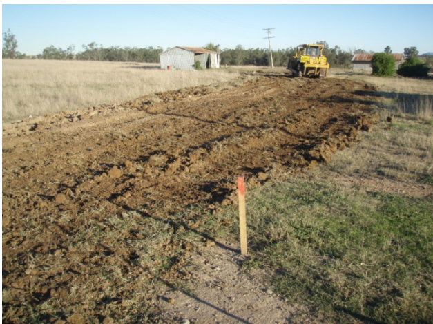
Figure 21. Subsidence crack remediation
