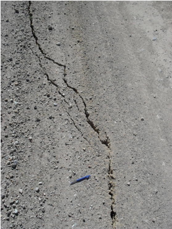
Figure 20. Subsidence cracks, Longwall 4
