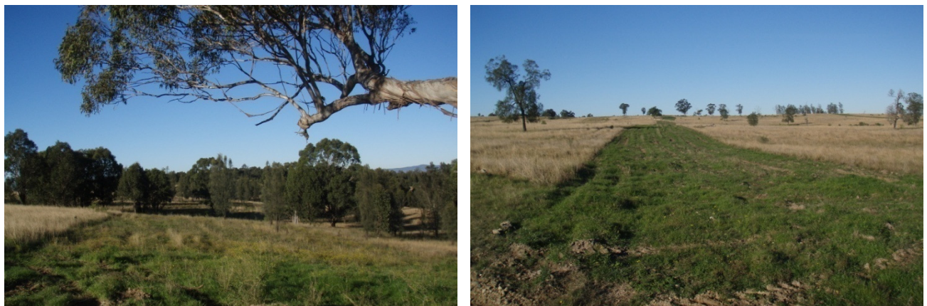
Figure 15. Subsidence crack remediation
