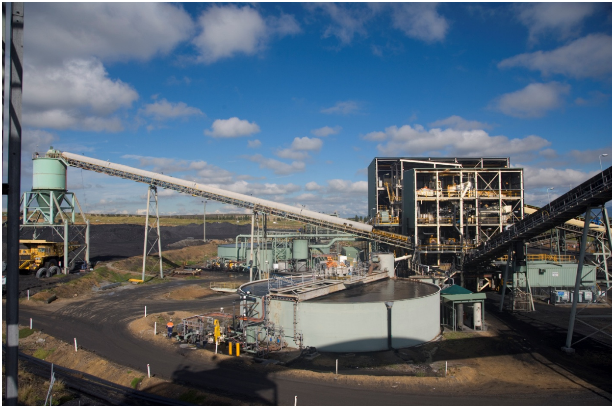
Figure 2. Coal Handling Preparation Plant
