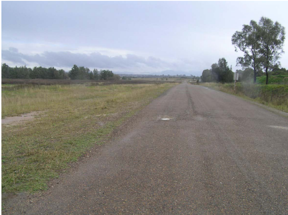
Figure 15: Sealed section of Brunkers Lane.
