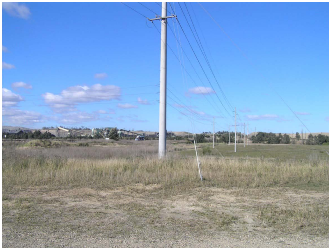
Figure 9: Photograph looking east along New England Highway road reserve.
