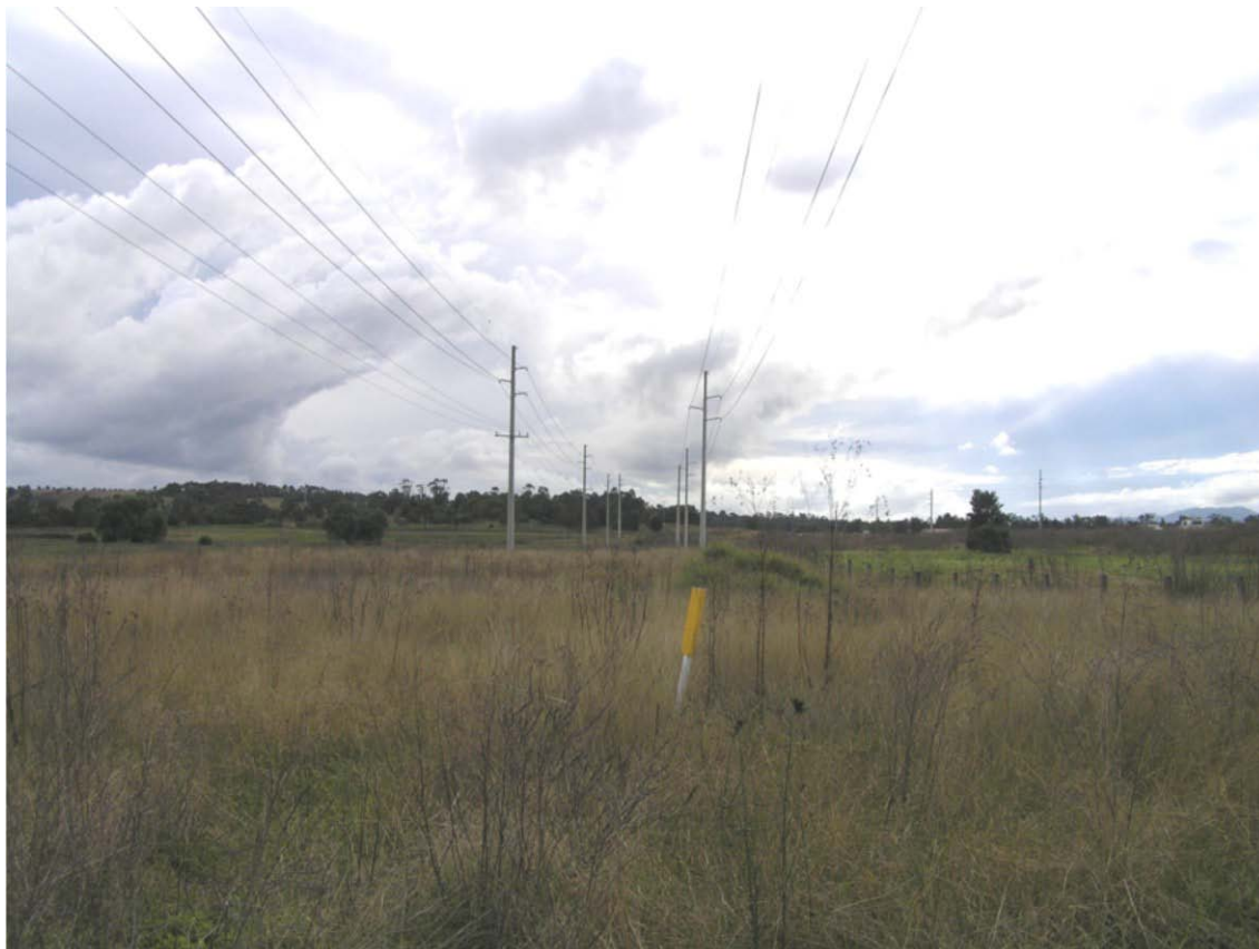
Figure 10: Photograph of Powertel cable and high voltage power lines in New England Highway road reserve.
