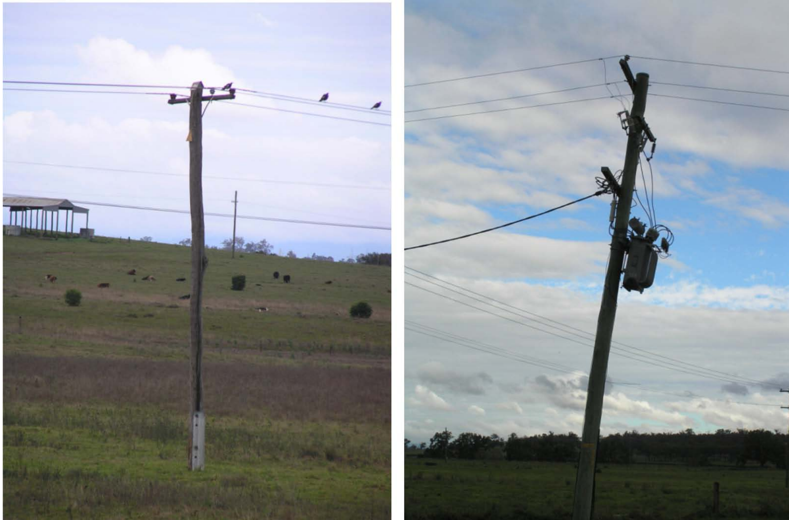
Figure 13: Photographs of single pole structures on local electricity lines.
