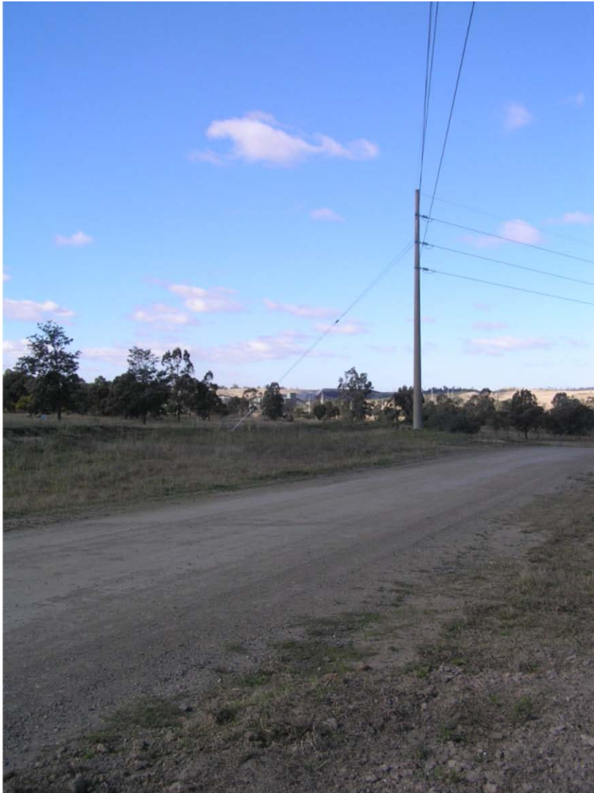
Figure 16: Unsealed access road on Macquarie Generation lease.
