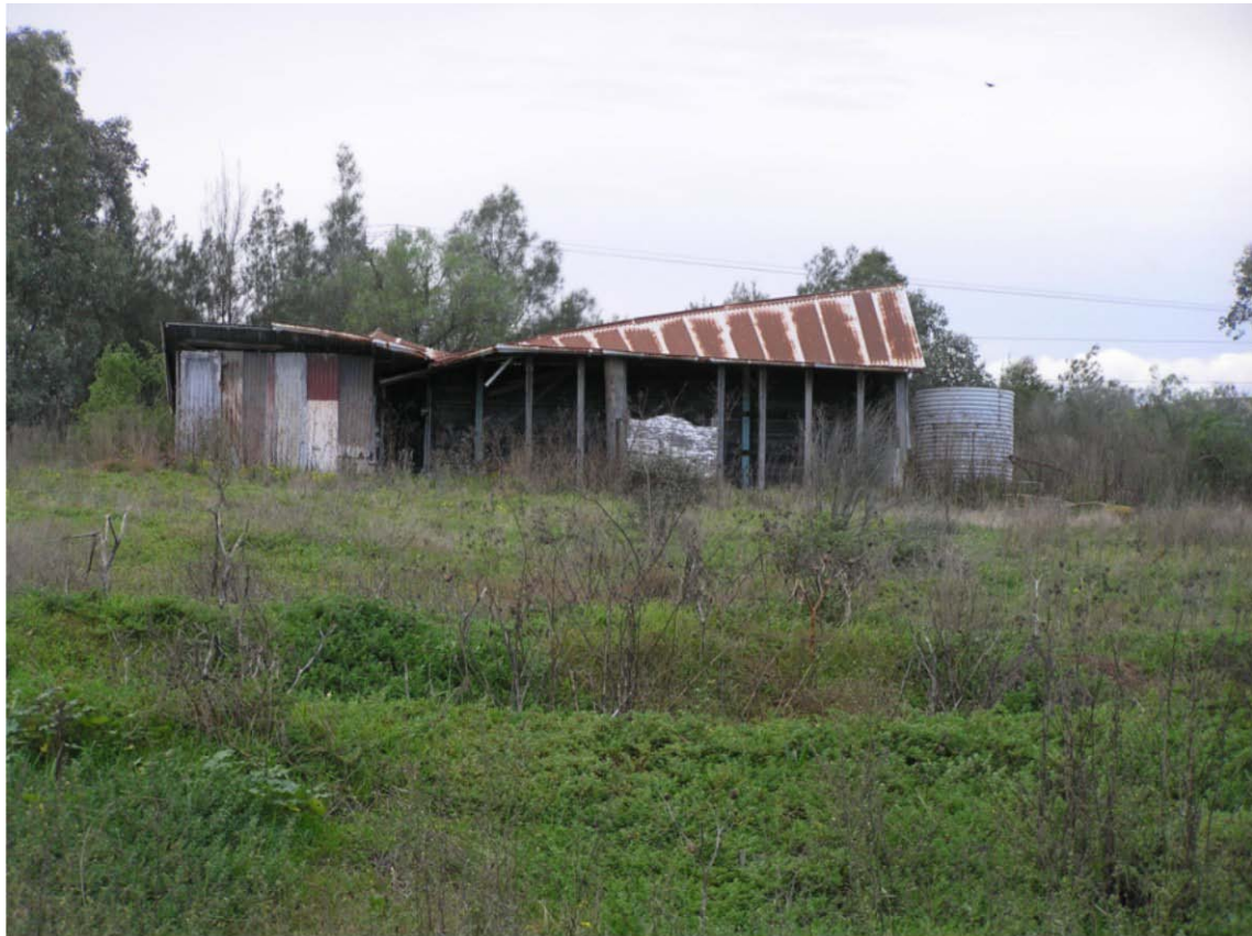
Figure 22: Disused shed beyond the northern end of Longwall 8.
