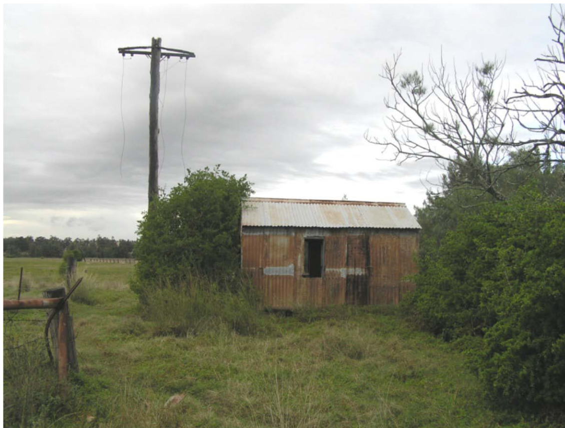
Figure 21: Disused pump shed adjacent to Bowmans Creek.
